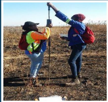
DRILLING OF WATER BOREHOLES
