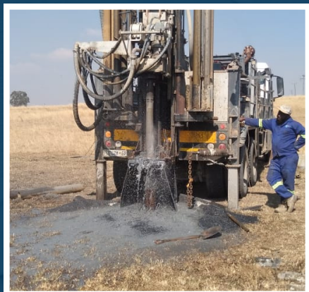
DRILLING OF WATER BOREHOLES
