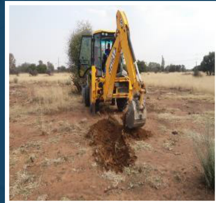
DRILLING OF WATER BOREHOLES
