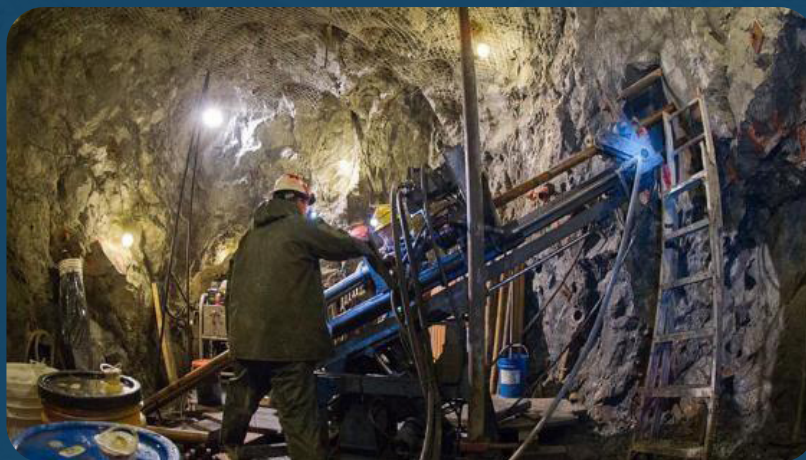
DRILLING OF WATER BOREHOLES
