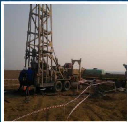
DRILLING OF WATER BOREHOLES
