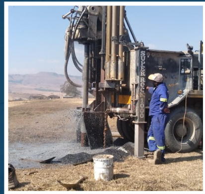
DRILLING OF WATER BOREHOLES
