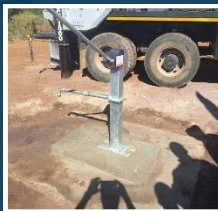
DRILLING OF WATER BOREHOLES
